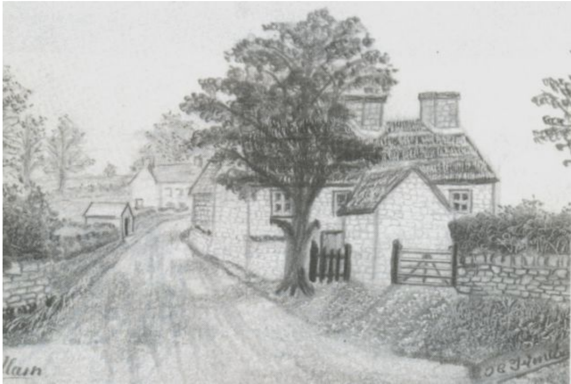
Maudlam Farm which was demolished circa 1959. Sketch by O.G. Trinder from "Sketches of Old Kenfig & District"[1992] with the kind permission of The Kenfig Society *.
