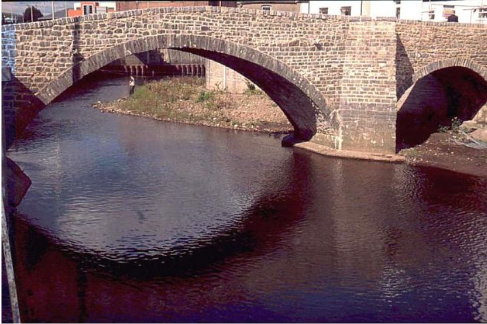
The Old Bridge (photo by Cyril James)
